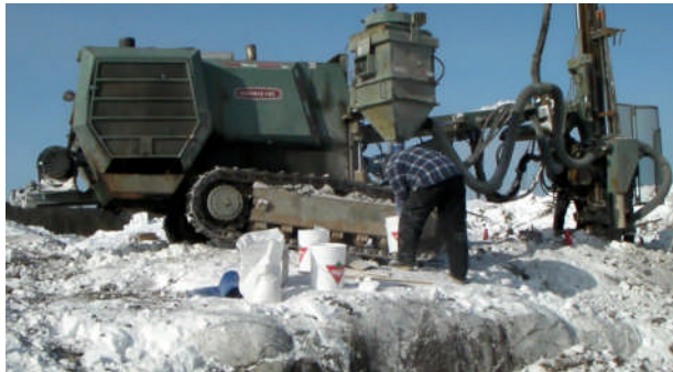
Drilling and sampling Production holes (Feb. 15 th , 2015)
